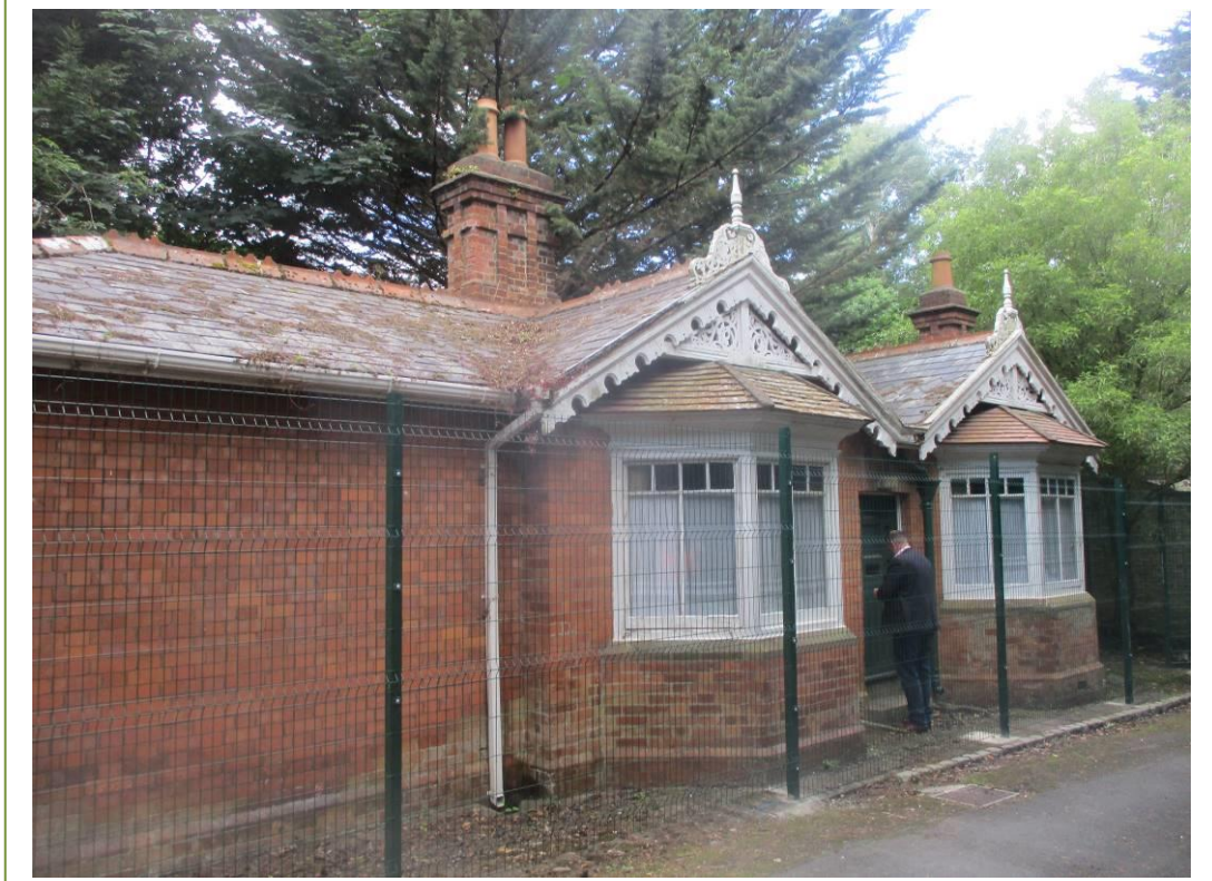
Red Brick Gate Lodge
