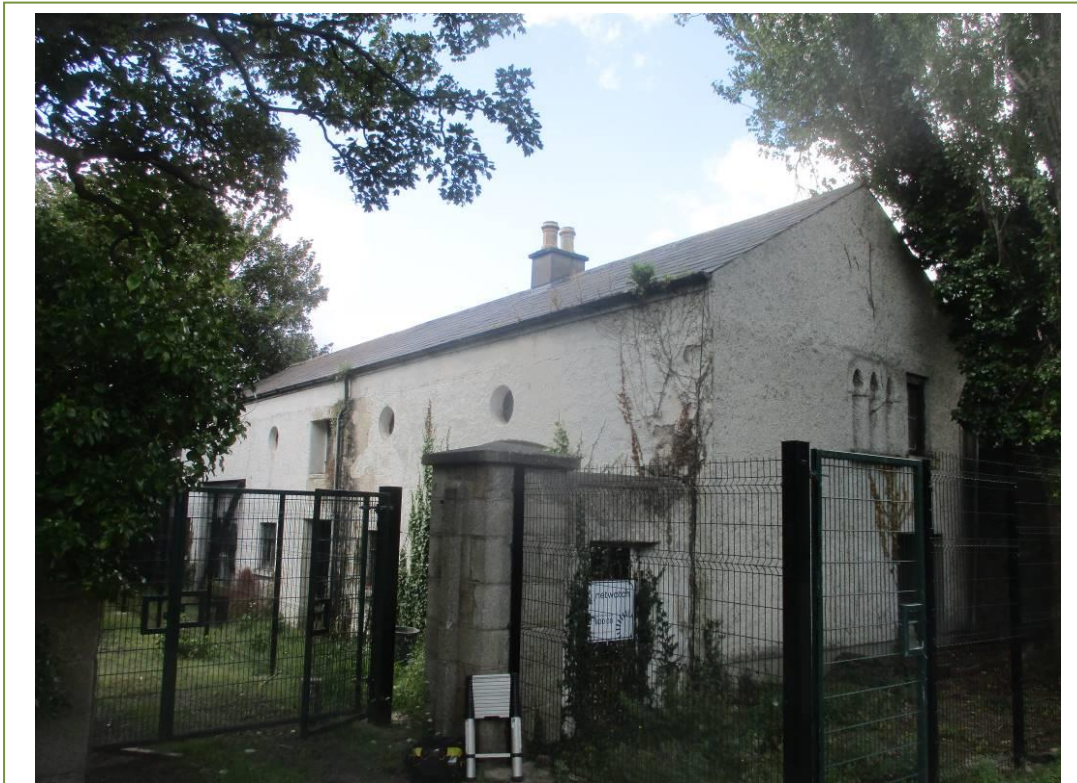
Natural slates on the roof of the stable block
