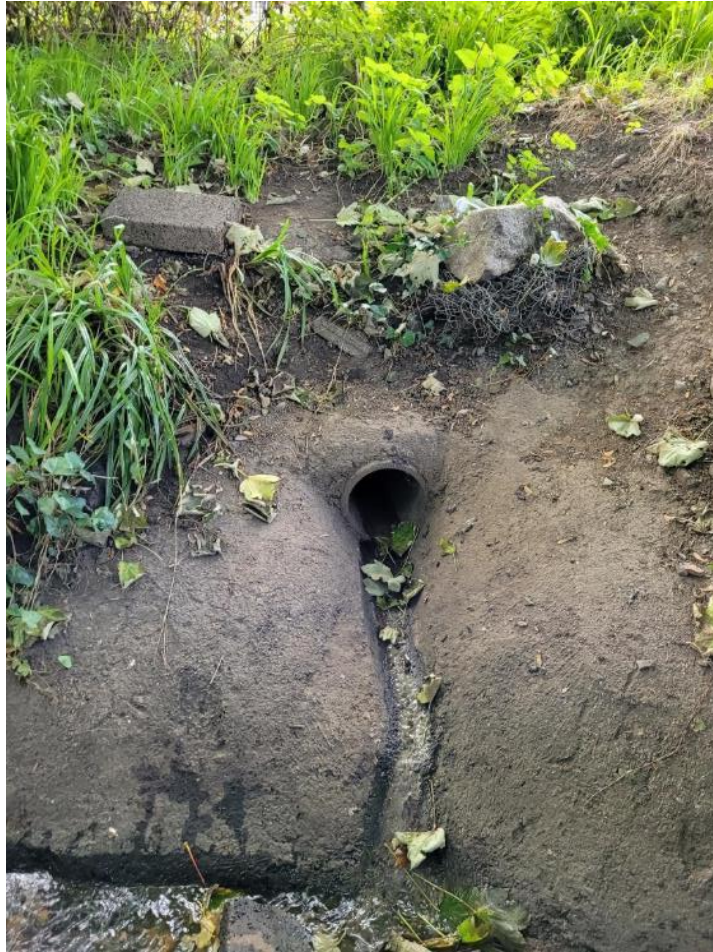
Figure G Site 2 - Storm drain adjacent to bridge
