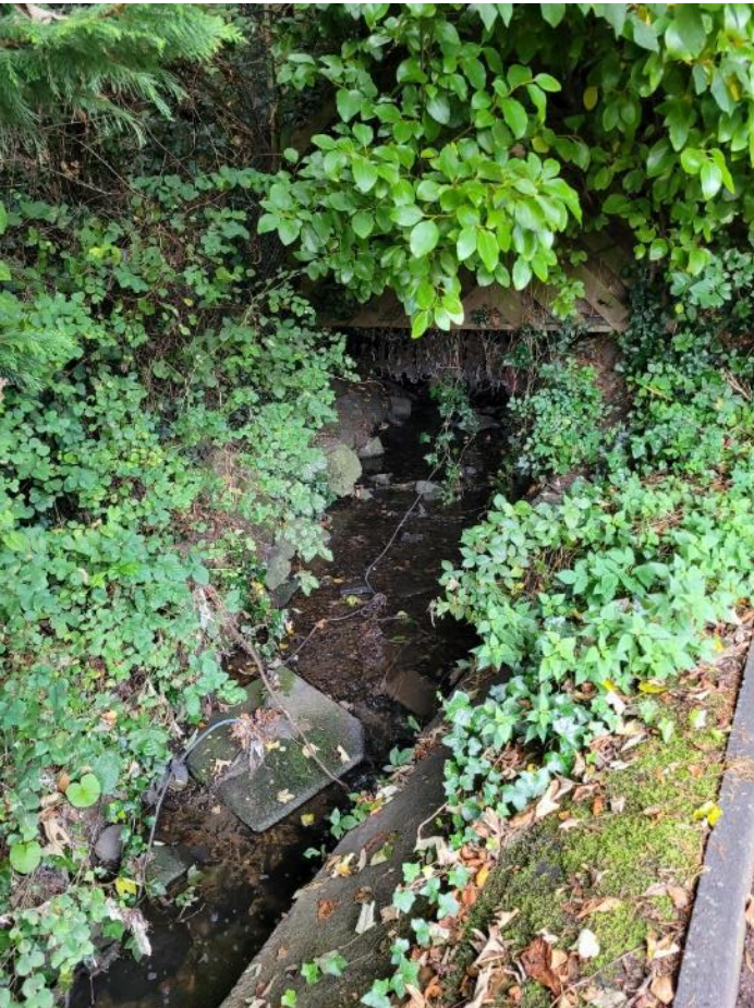
Figure A Site 1 - Facing Upstream
