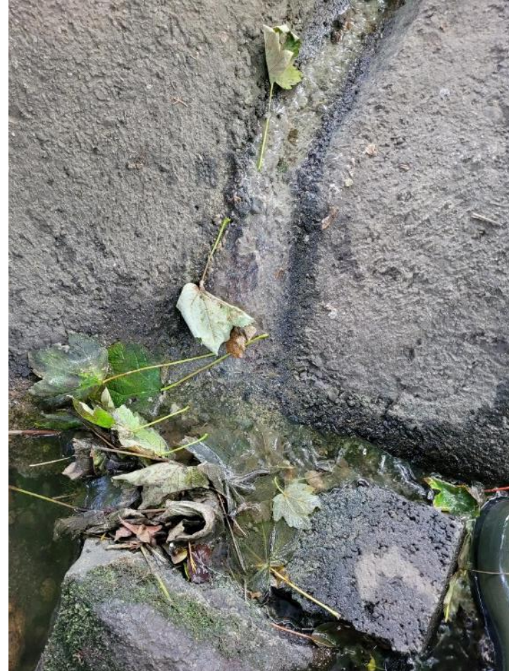
Figure H Site 2 - Sewage fungus at base of drain
