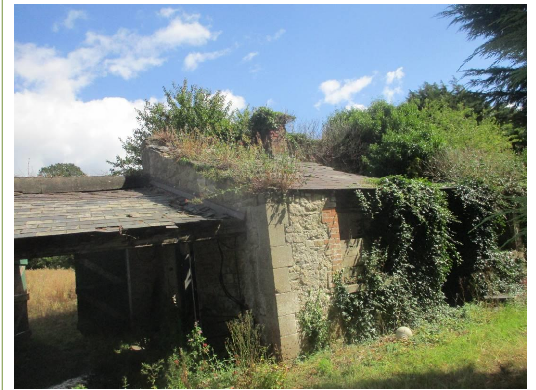
Rear derelict buildings
