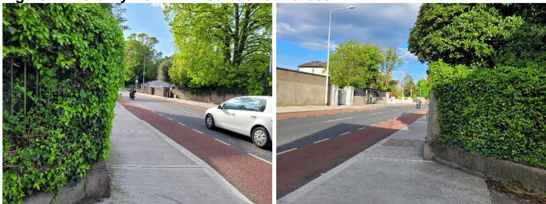
Figure 3: Visibility from 2.4m setback at Dalguise House Access
