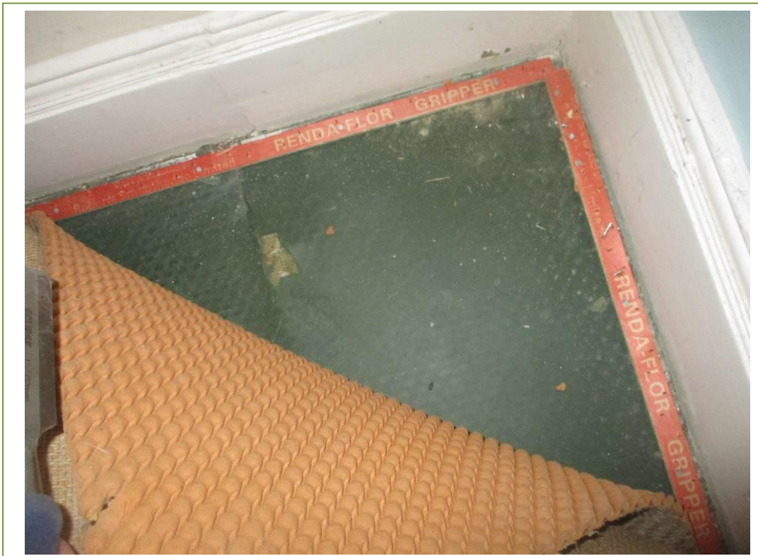
Floor covering in the 1 st floor bedroom in the main house
