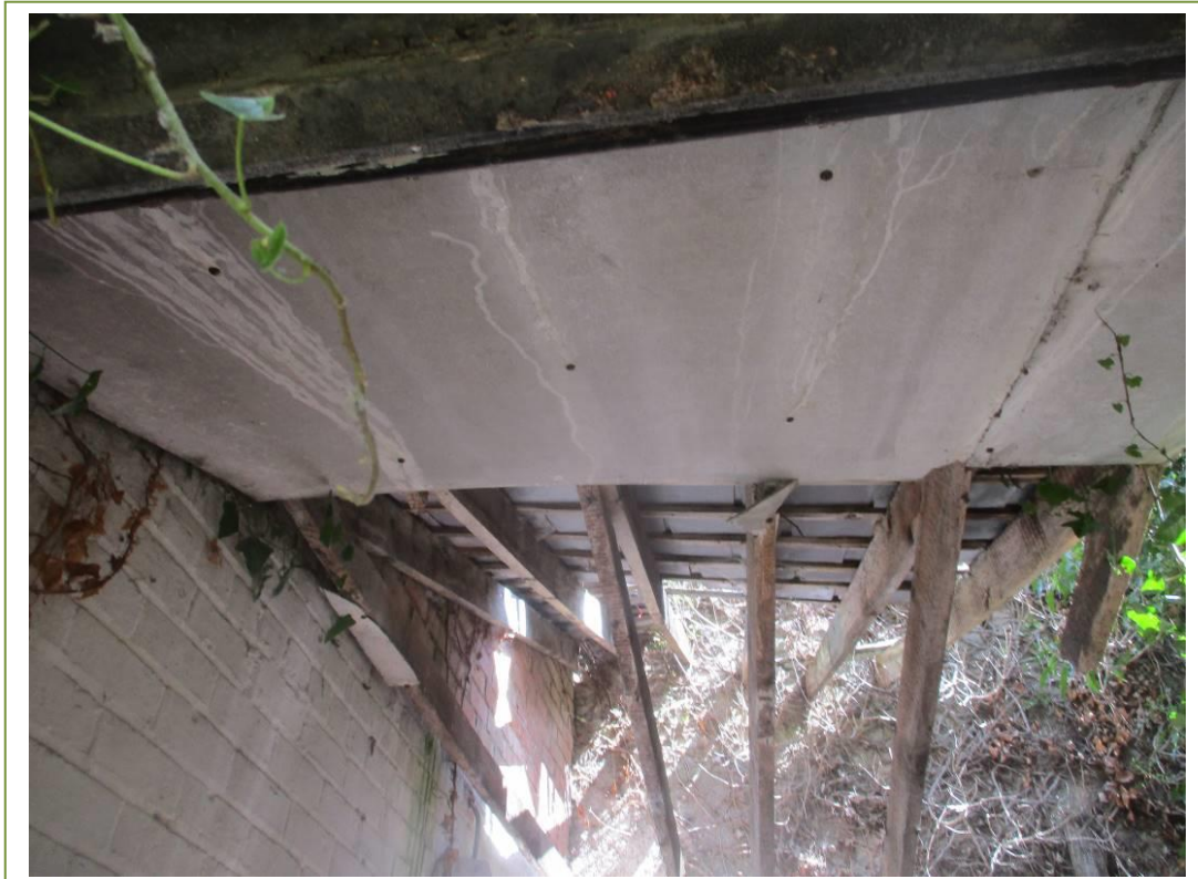
Asbestos cement ceiling board in the rear derelict building
