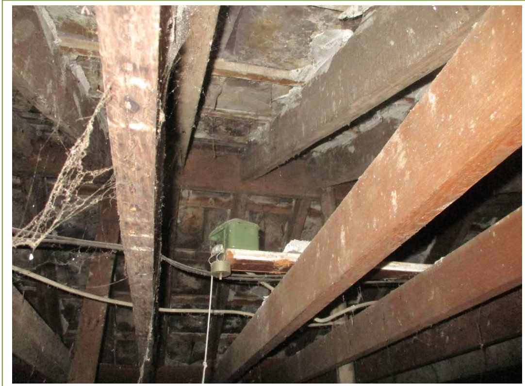
Slates on the main roof
